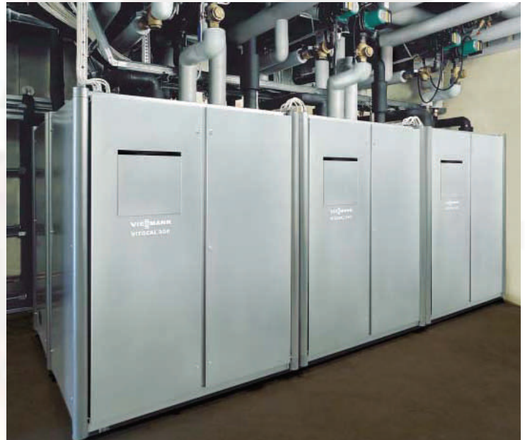
640kW Local Heating System by Viessmann
